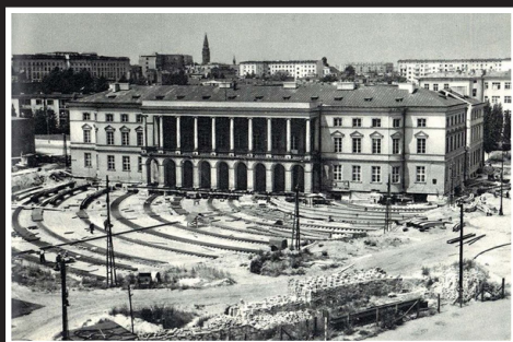
Lubomirski Palace being moved to its new location.
